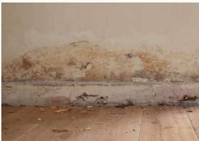
**Damp** occurs when water finds its way into a property, usually from outside. This can happen in a few ways such as damaged gutters, broken roof tiles or even through the foundations of your home, which is called **rising damp**. Damp may also be caused by an internal leak. It should be easy to identify as a dark, wet patch that may also cause flaky plaster and a pungent smell.
